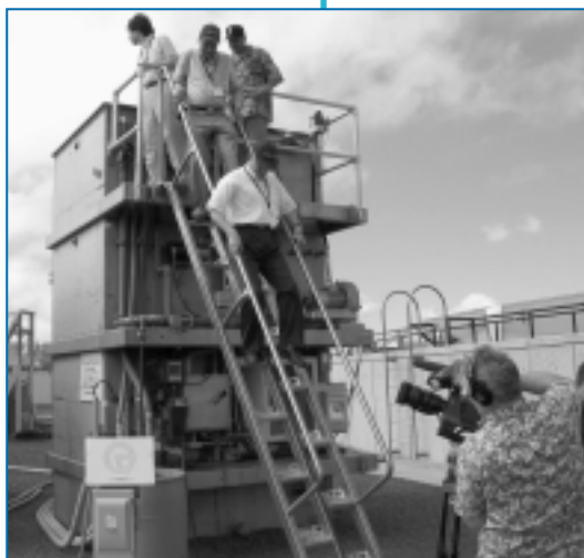
Symposium attendees take a look at the Enviroquip 0.04-micron, flat-panel membrane bioreactor while touring the Honolulu Membrane Bioreactor Pilot Study Site, located at the Honouliuli Wastewater Treatment Plant and sponsored by the Honolulu Board of Water Supply.
